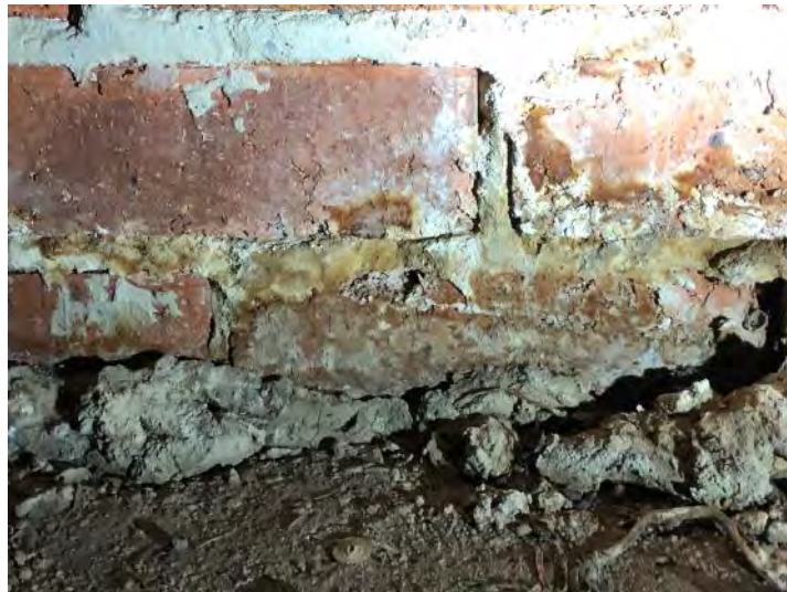
Example of moisture penetration/water seepage to bottoms of a few walls.
