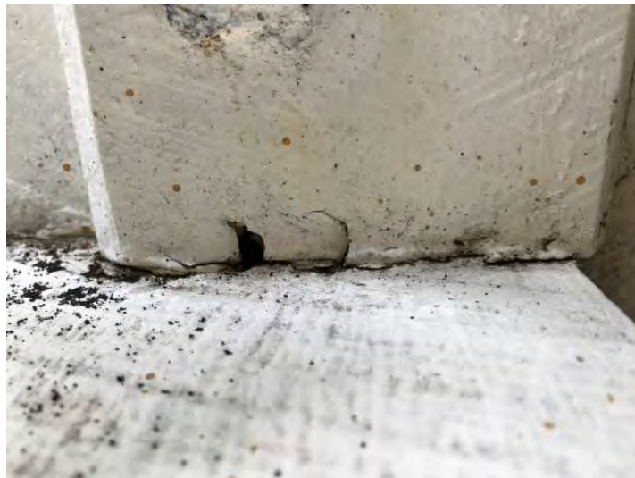
Example of Wood Rot/Weathering to bases of newel posts.
