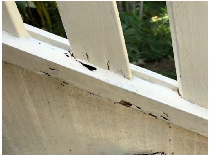
Example of woodrot to handrails/barriers.
