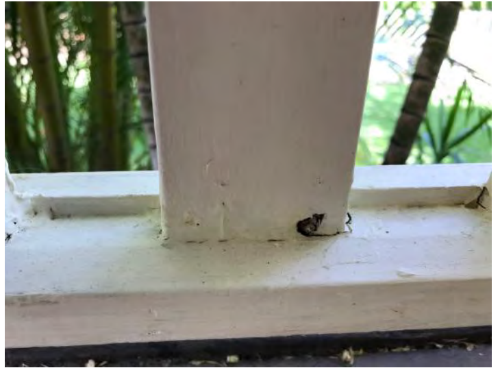
Example of Wood Rot to bottoms of a few Balusters.
