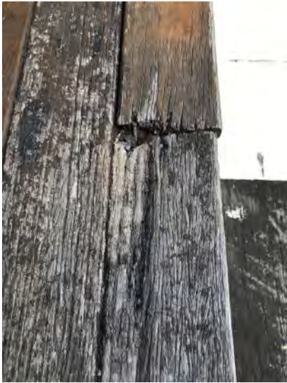
Example of Wod Rot to timber decking at top of Stairs.
