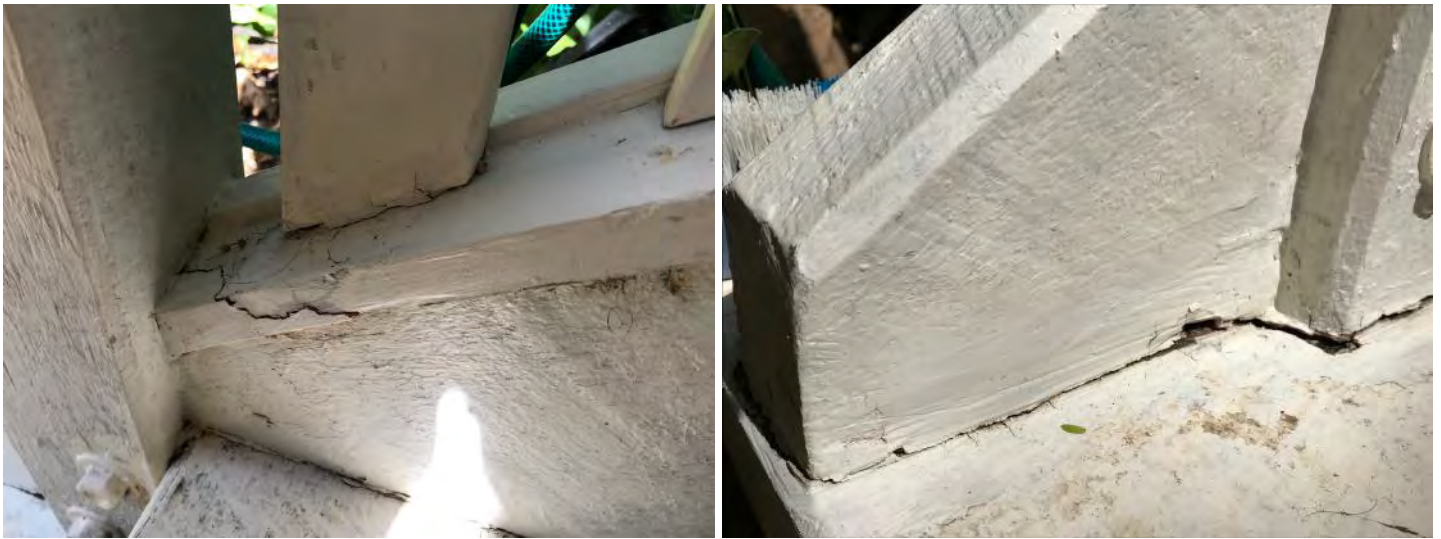
Example of Wood Rot to parts of Handrails/Barriers.
