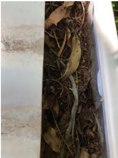
Example of gutters needing to be cleaned.
