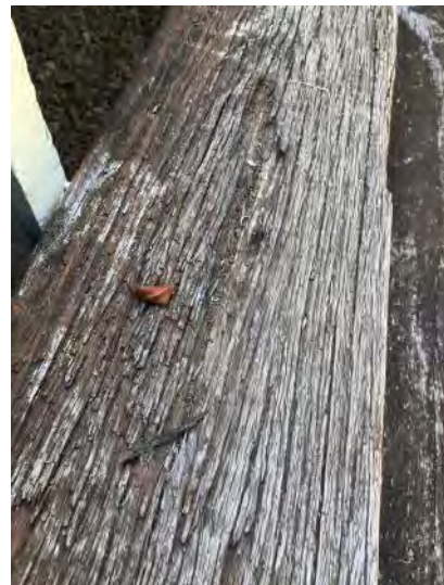
Example of heavily weathered timber treads.
