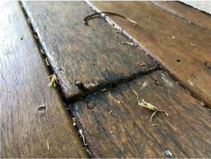
Example of loose and weathered decking timbers.
