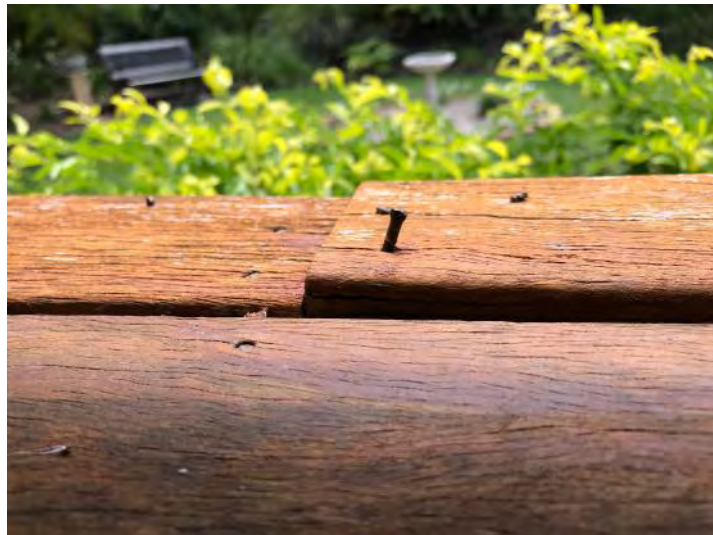
Example of weathered/loose decking.
