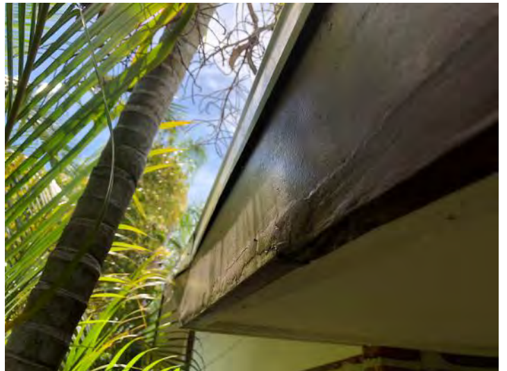
Example of Wood Rot to Western end Fascia.
