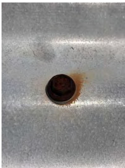
Example of rusty roof screws.
