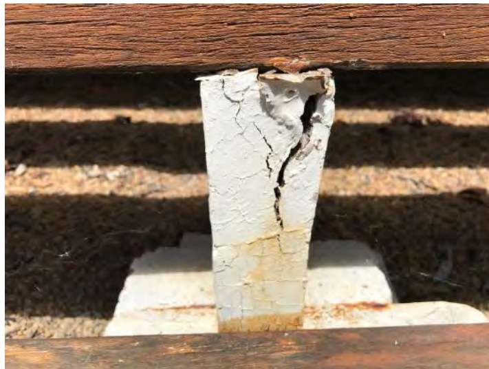
Example of split/weathered middle stringer.
