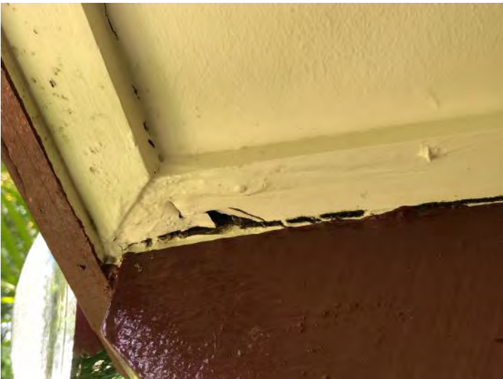
Example of water damaged soffit mouldings.
