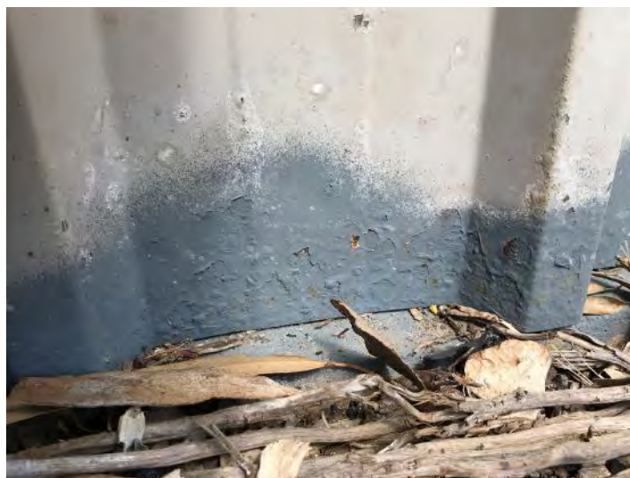
Example of rusty sections of wall sheeting.
