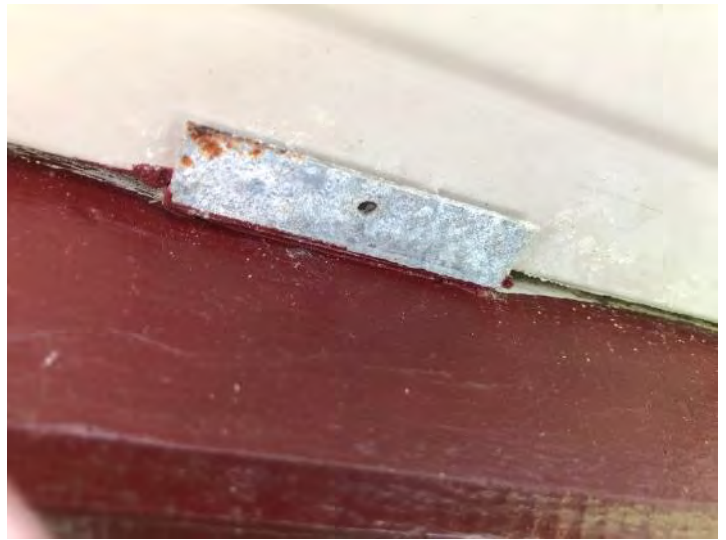
Example of rusty/corroded gutter brackets.
